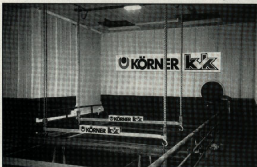
Figure 2. Enclosed pre-treatment unit; no personnel allowed inside the enclosure
